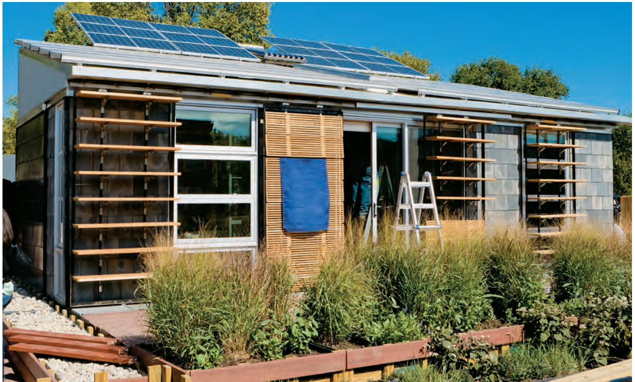
This small, energy-efficient modern house uses PV panels for power. Energy is conserved with energy-efficient appliances, extra insulation, a light-colored roof to deflect heat, and louver-shaded windows.
