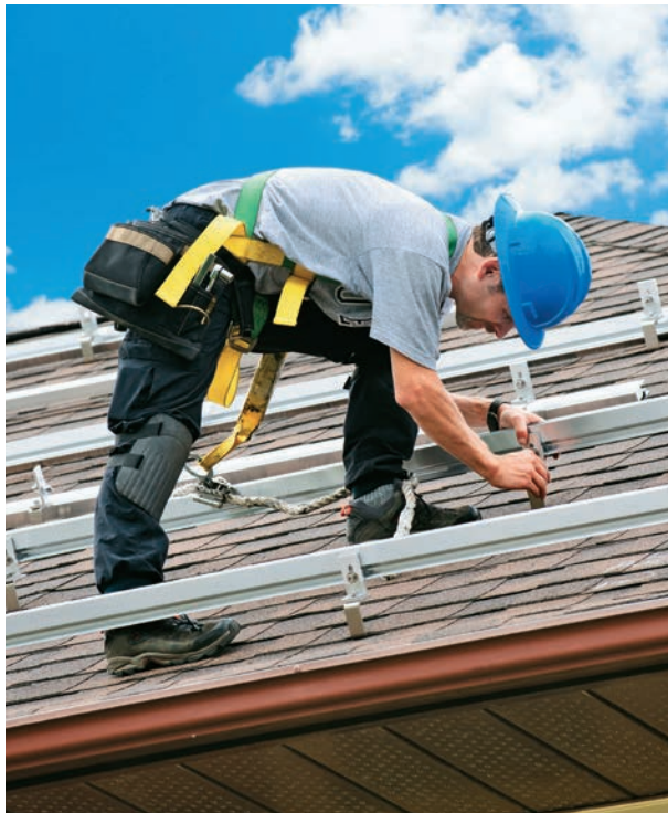
Wear a proper safety harness when working on a steep roof.
