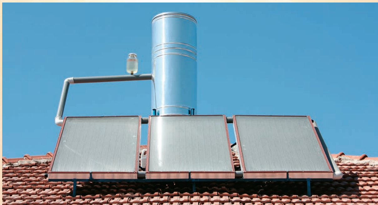
Thermosyphon tanks must be above the level of the collector in order for the movement of water by thermosyphoning to occur.
