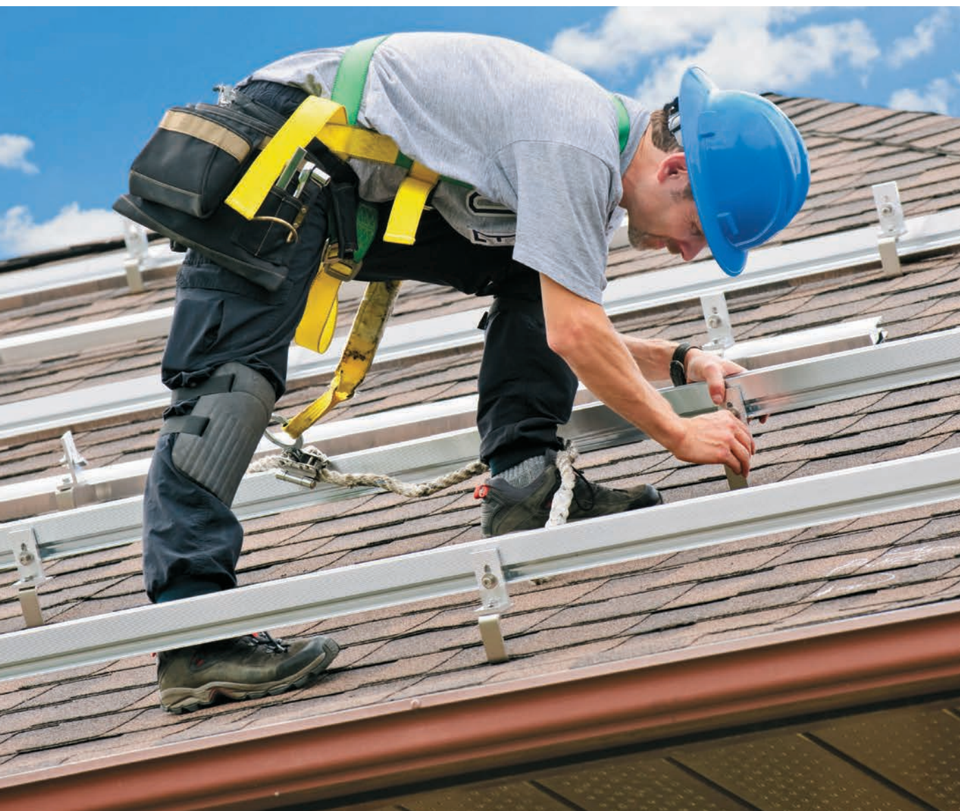
A system of mounting rails is attached directly to the roof framing members with lag screws.
